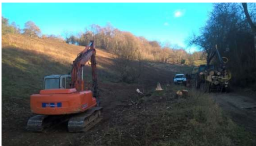
Contractors working at the bottom of the Terraces.
